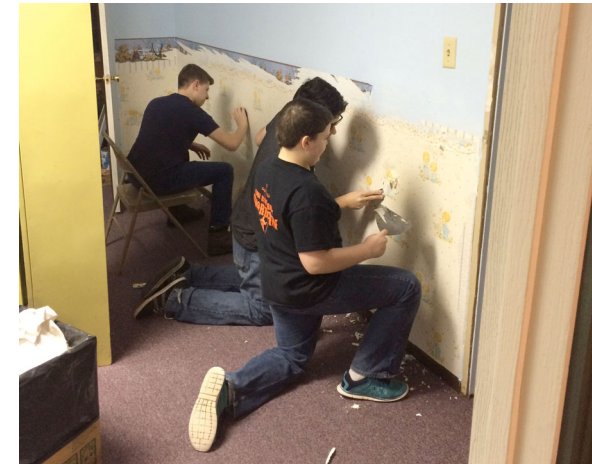
Operation: Declutter, Phase 2 — wallpaper removal for new paint, with Caleb, Kieran, and Tyler!
